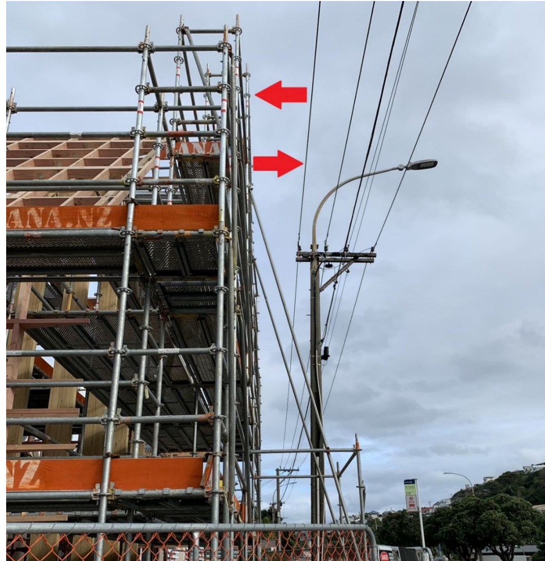
Network lines and scaffolding
