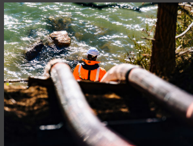
Ducting down the bank at Portobello
