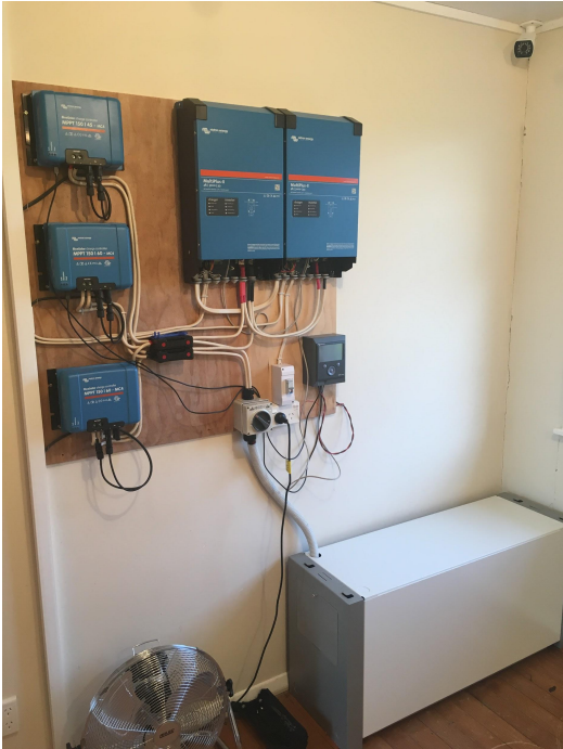
Solar PV/Battery Controller
