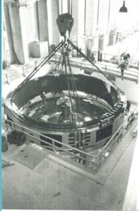
Aviemore stator being lowered into place
